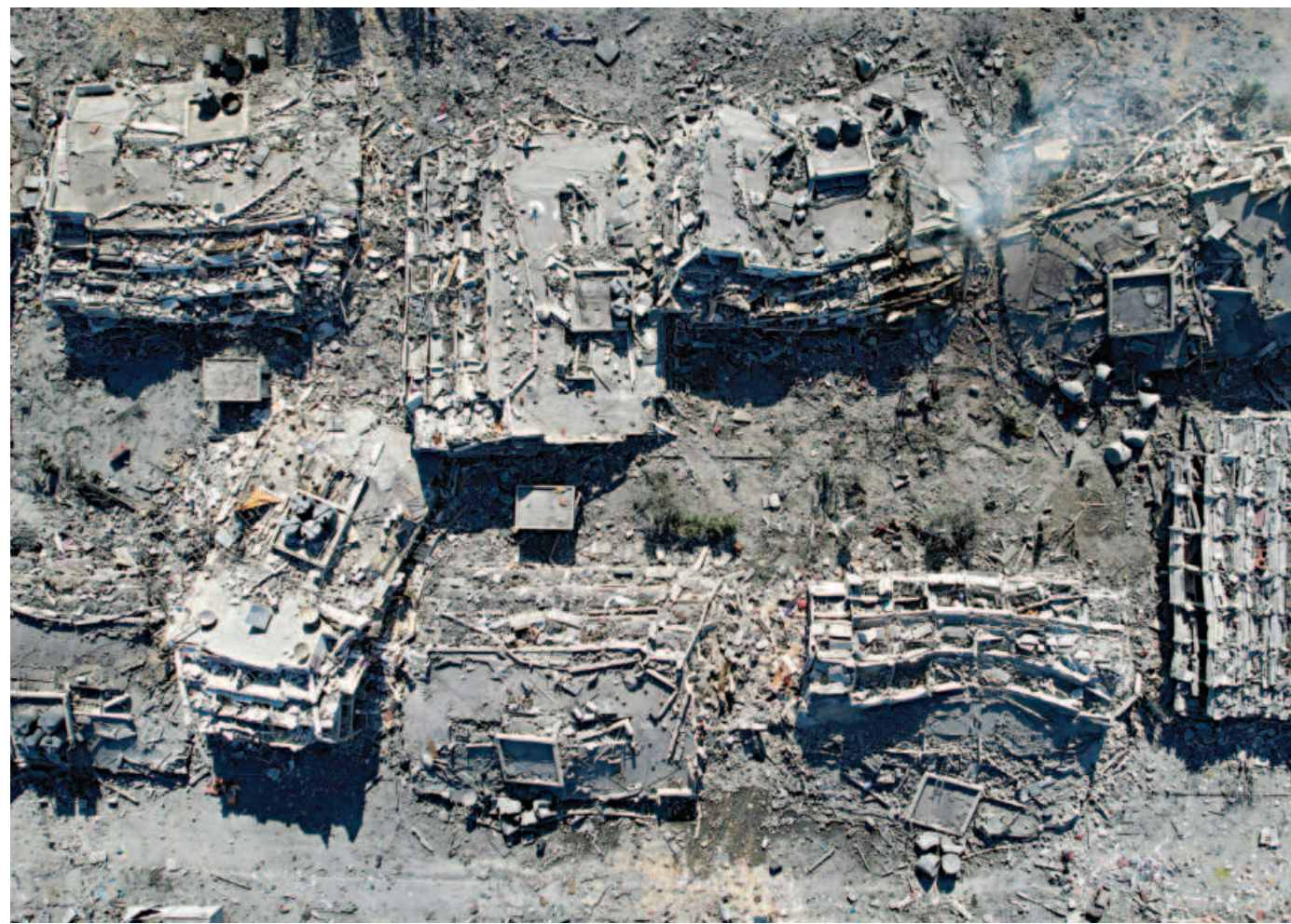
A view of residential buildings destroyed in Israeli strikes in Zahra in southern Gaza City yesterday.
