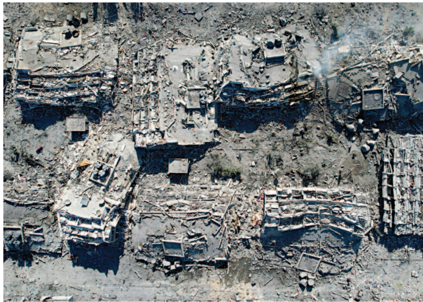
A view of residential buildings destroyed in Israeli strikes in Zahra in southern Gaza City yesterday.
