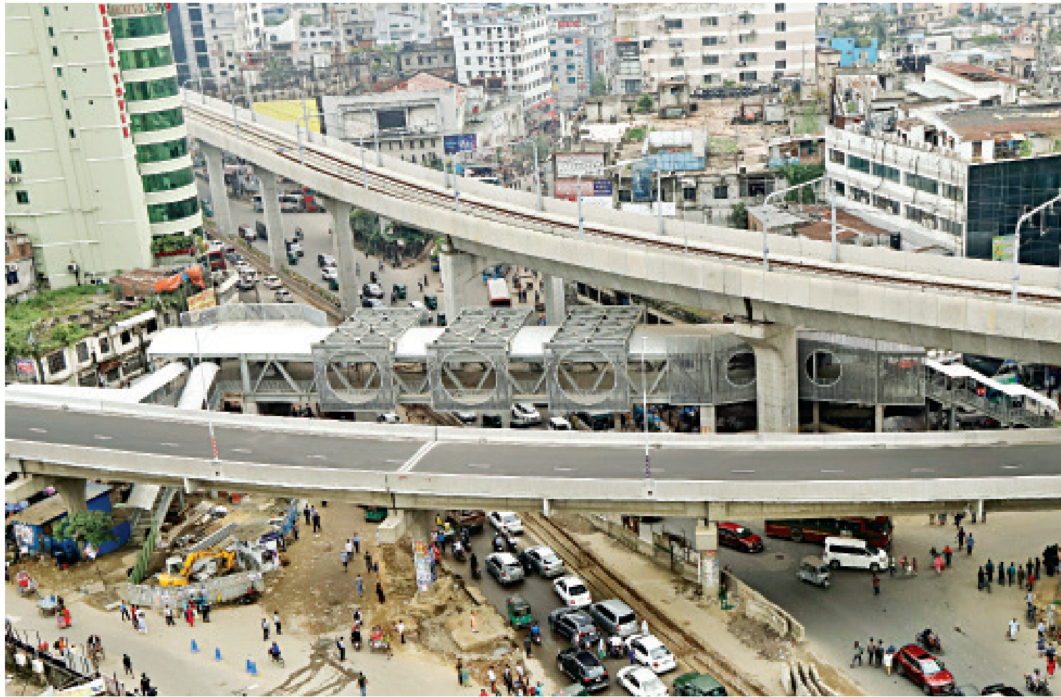
After one and a half years of closure due to construction work of the Dhaka Elevated Expressway, the Farmgate footbridge will be inaugurated today. Being the first of its kind, the bridge, designed in the pattern of the parliament building, was built at a cost of Tk 20 crore. It will have escalators and lifts at both ends for pedestrians. The photo was taken yesterday.
