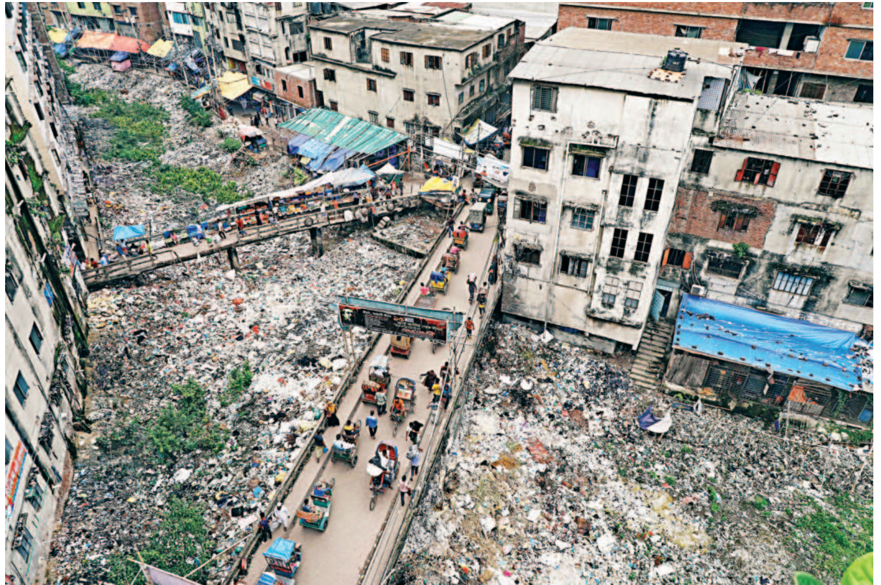
The Shuvaddya canal in Dakshin Keraniganj has literally been turned into a dumping ground by sweatshops and traders of kitchen markets, leaving no room for water to flow. The photo was taken yesterday. PHOTO: PALASH KHAN
