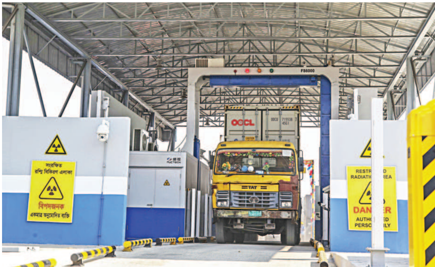
Currently there are seven container scanners at the Chattogram port, all being used to look into imports.
