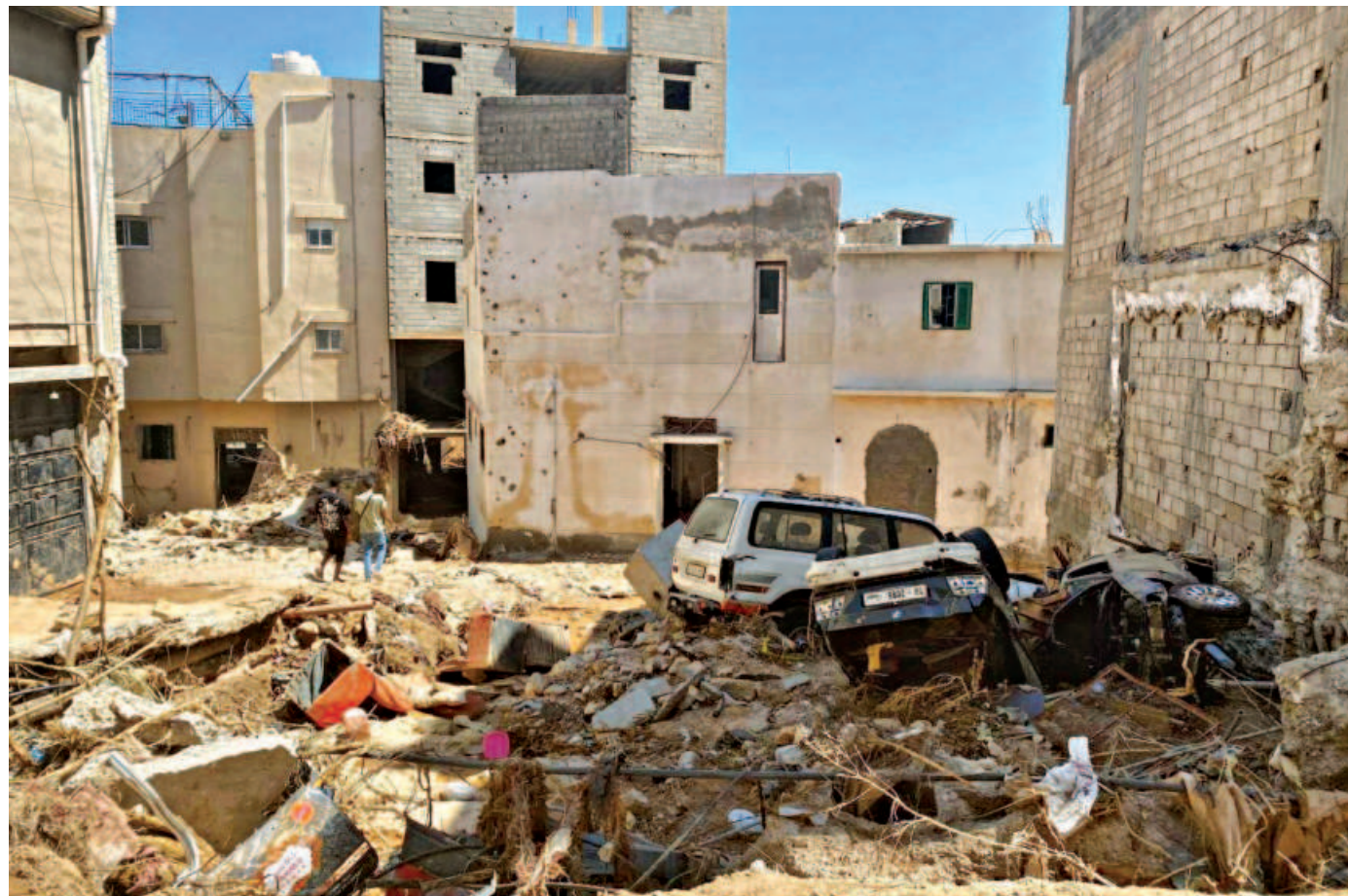
People walk amidst the wreckage, in the aftermath of the floods in Derna, Libya yesterday. The floods were caused by hurricane-strength Storm Daniel, compounded by the poor infrastructure in Libya, which was plunged into turmoil after a Nato-backed uprising toppled and killed longtime dictator Moamer Gaddafi in 2011.
