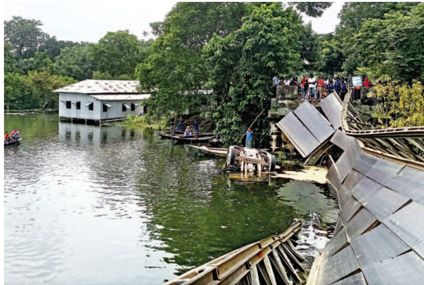
A Bailey bridge in Tangail's Delduar upazila collapses early yesterday when a sand-laden truck was crossing it. This severed direct road communication between Delduar upazila and Tangail town.
