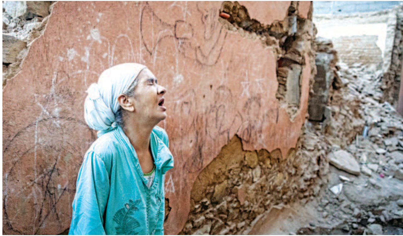
A woman standing in front of her earthquake-damaged house in the old city in Marrakesh yesterday. A powerful earthquake shook Morocco late Friday. PHOTO: AFP
