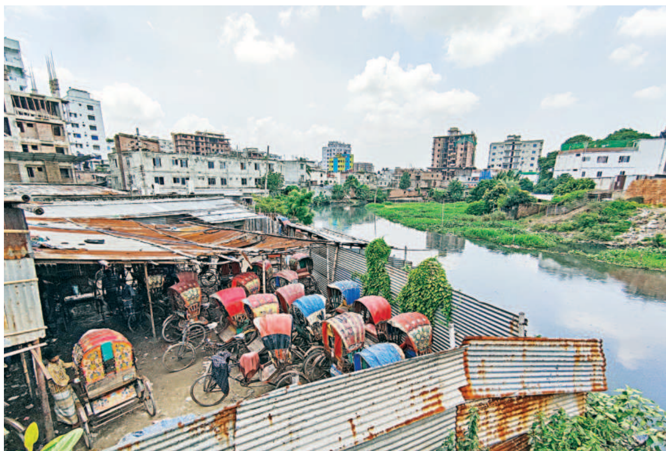
A rickshaw garage has been set up encroaching upon the Kalyanpur canal in Goidertek area of the capital's Adabar. Illegal structures like this obstruct the flow of water in the canal, leading to waterlogging in many parts of the city during monsoon. The photo was taken recently.
