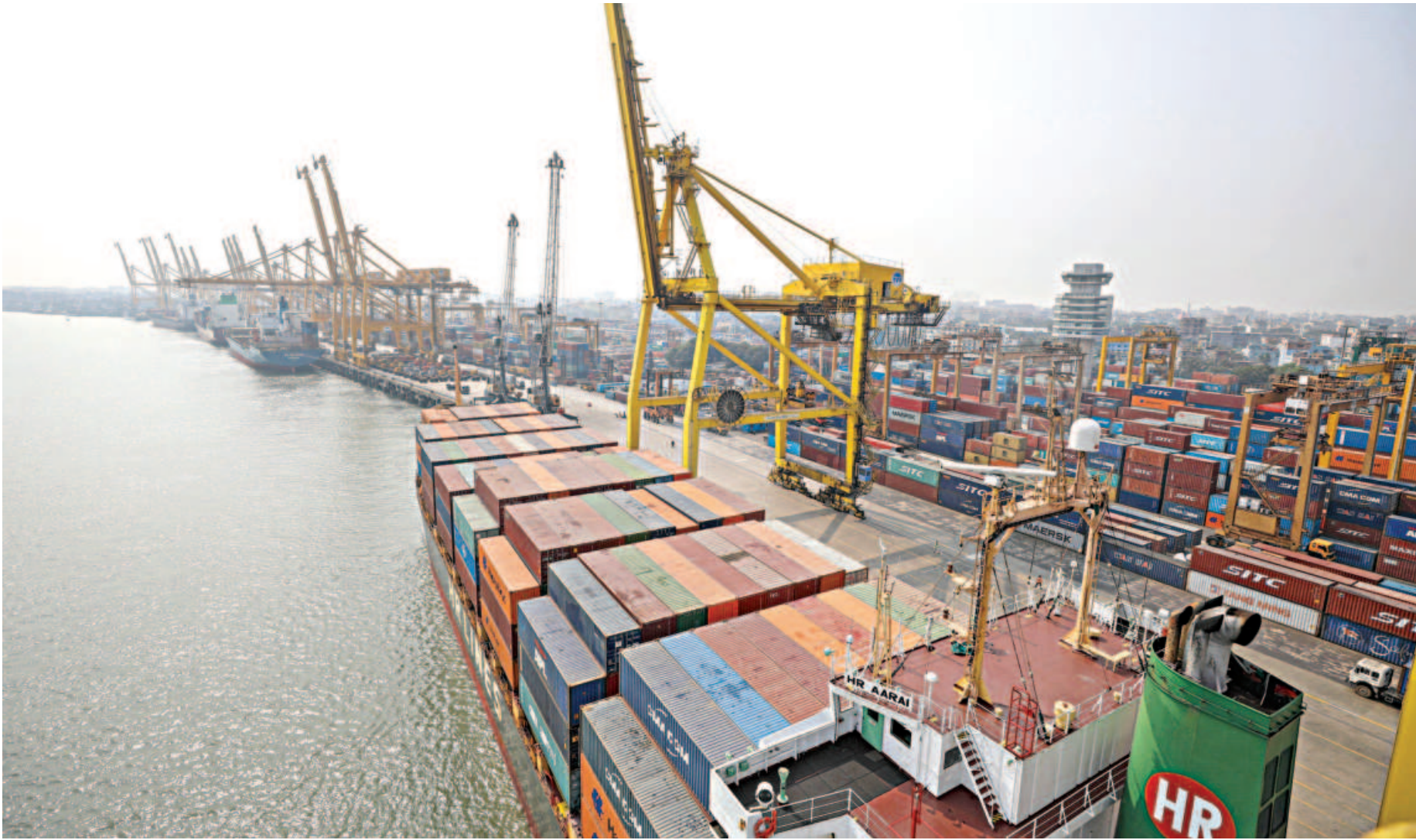
A partial view of the premier seaport of the country in Chattogram. Six incidents of theft and piracy took place in vessels arriving at the port in the six months to July this year.
