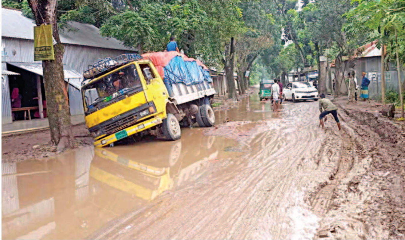
This important road, stretching from Sakhipur to Sagardighi in Tangail, is in an appalling state due to lack of renovation work for long, making it difficult for vehicles to cross it. The photo was taken recently.
