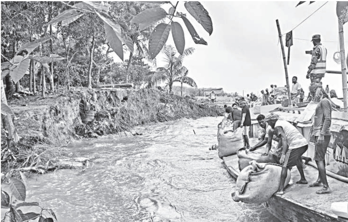
Water Development Board officials deploy geo bags as the swelling Padma erodes its banks in Manikganj’s Harirampur upazila. The river has already devoured 12 homesteads, arable lands, and a local primary school. The photo was taken yesterday.
