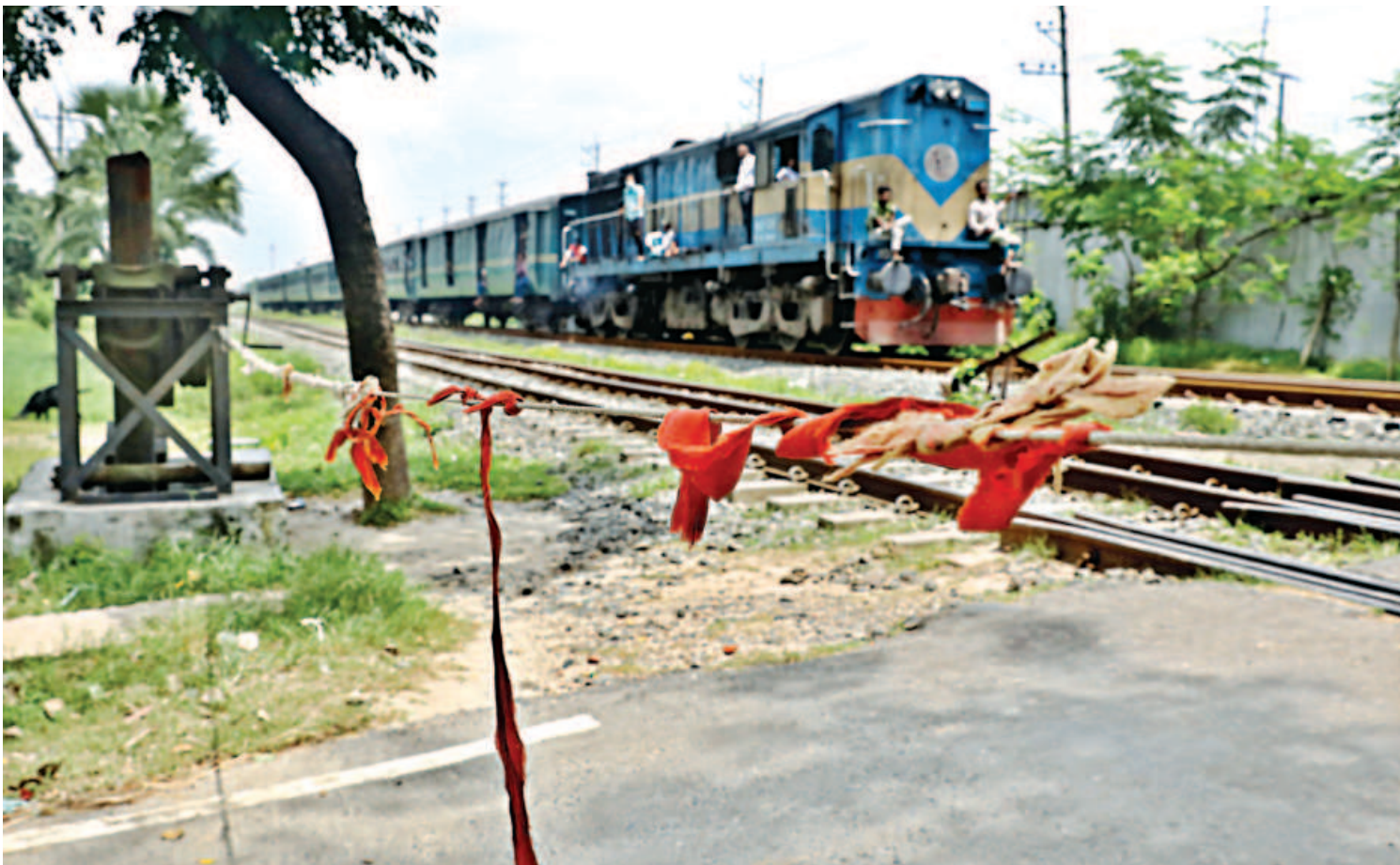
Since there is no gate to block traffic when trains approach, the gatekeeper ties a rope at the level-crossing in Hyderabad area of Gazipur. Strips of red cloth are attached to the rope to increase visibility. A proper barrier is needed to make the level-crossing on the busy street safer.
