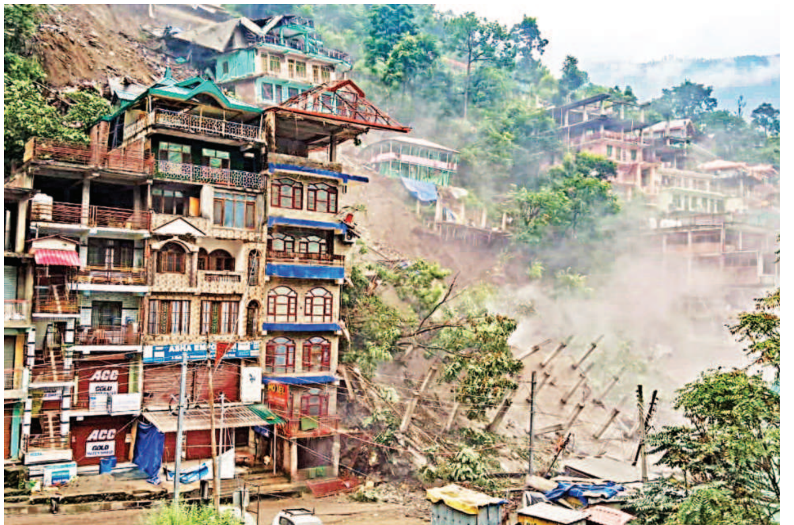
Several buildings collapse after massive landslides following heavy rainfall at Kullu's Anni town, in India's Himachal Pradesh state yesterday. No one was hurt in the landslide as residents had been moved out of the area because it was deemed unsafe. PHOTO: AFP
