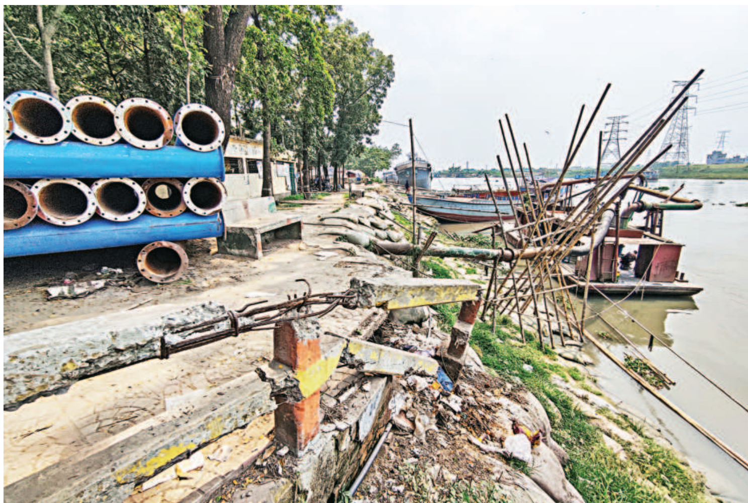
Constructed to serve pedestrians and prevent erosion, the walkways along the river Turag dilapidate as large vessels continue to dock its bank illegally. The photo was taken recently from the capital's Gabtoli.
