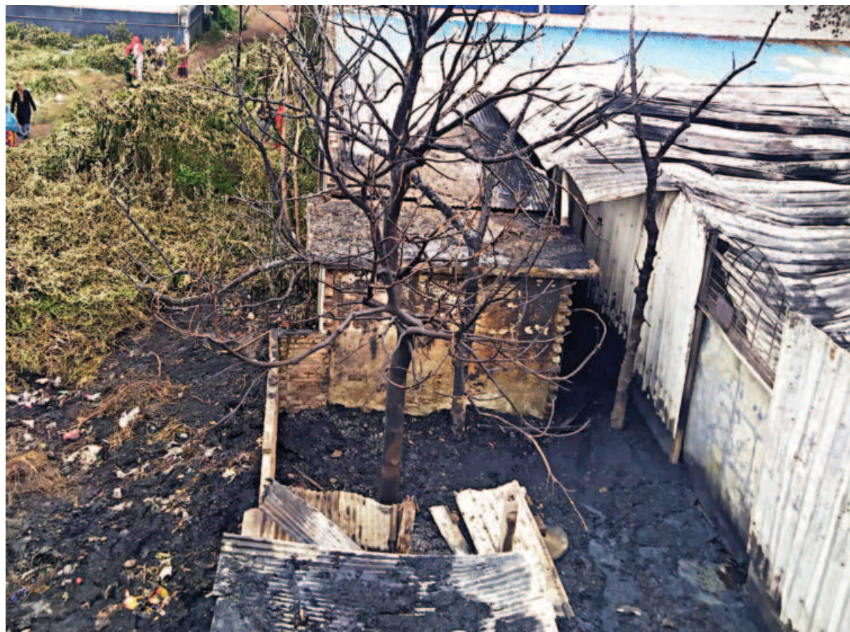
The charred remains of a chemical warehouse and its front area in Keraniganj's Gadarbagh, after a massive fire ripped through it early yesterday. Five of a family died and at least 15 others were injured as the fire gutted two tin-roof houses adjacent to the warehouse. According to fire service officials, flammable chemicals caused the fire to spread, while the source of the flame is yet to be confirmed. Meanwhile, locals alleged the warehouse was built illegally by a chemical trader from Dhaka's Churihatta.
