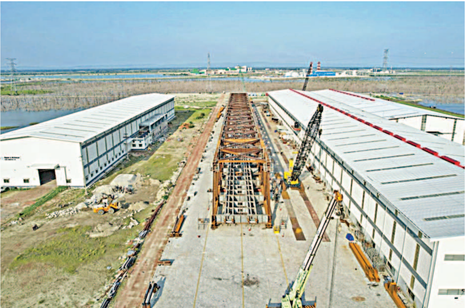
A prefabricated steel structure to be used in the Bangabandhu Sheikh Mujib Railway Bridge is seen under construction at a manufacturing facility of McDonald Steel Building Products Limited.
