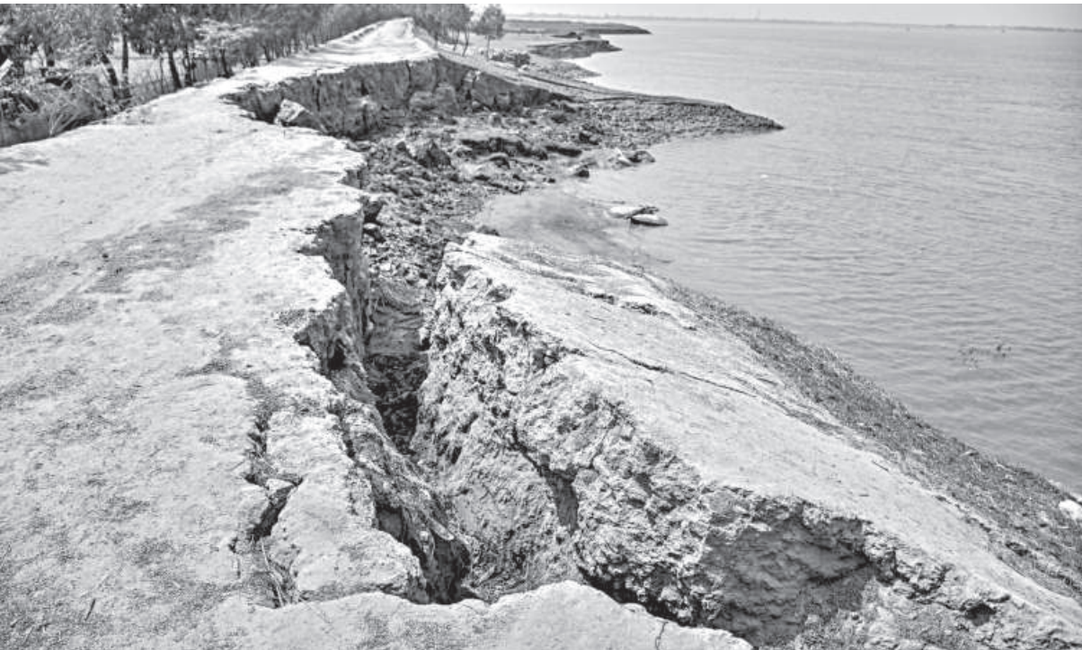
Around 20,000 people hailing from Khulna's Dacope upazila lose their homesteads and croplands to erosion as embankments constructed around 60 years ago remain unrepaired. While locals tried their best to salvage whatever they had by deploying geobags, the rising water levels following persistent rains kept damaging the banks. The photos were taken recently.
