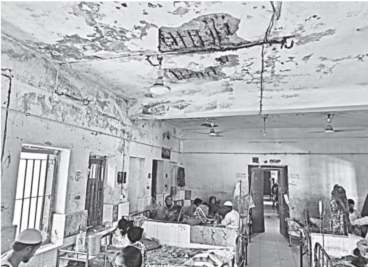
Four two-storey buildings of Baufal Upazila Health Complex in Patuakhali remain dilapidated for years due to a lack of repairs. The plaster falling off the ceiling has compelled the staff to wear helmets while on duty to save themselves from accidents. Meanwhile, rainwater enters the hospital through cracked walls, adding to the menace. A shortage of specialised physicians further exacerbates the patients' suffering.
