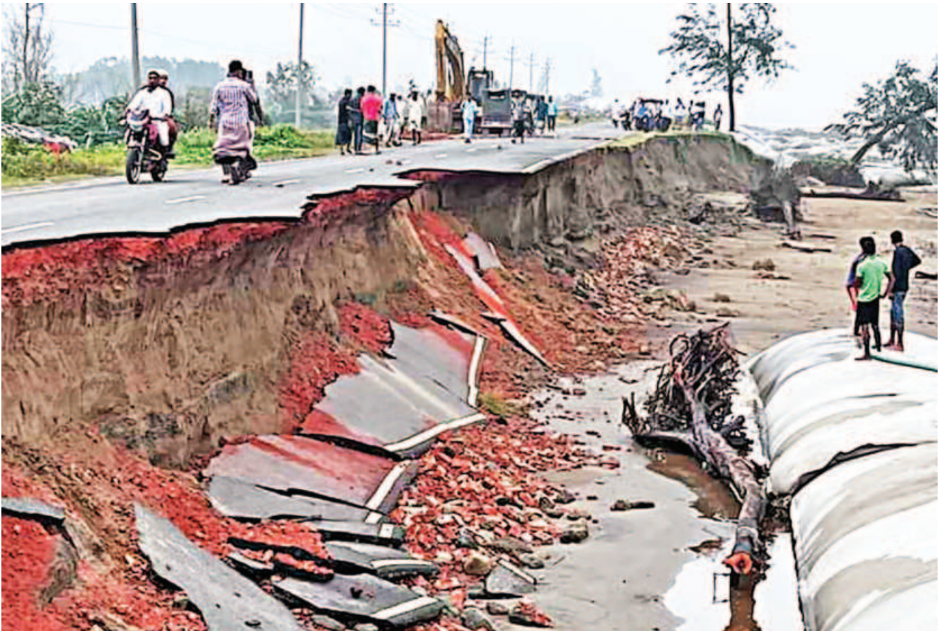
The erosion in some parts of the Marine Drive has taken a grave turn from Thursday, affecting at least 10 points in Teknaf. Around half of the 50-metre wide Marine Drive in west Mundardail area was washed away after geo tubes for protecting the road were torn apart by strong waves.
