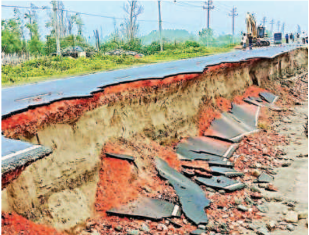
The erosion in some parts of the Marine Drive has taken a grave turn from Thursday, affecting at least 10 points in Teknaf. Around half of the 50-metre wide Marine Drive in west Mundardail area was washed away after geo tubes for protecting the road were torn apart by strong waves.
