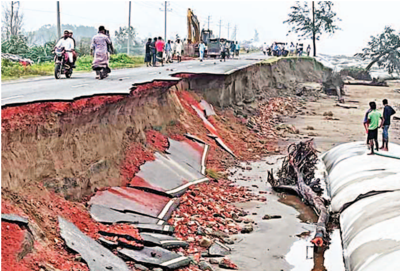
The erosion in some parts of the Marine Drive has taken a grave turn from Thursday, affecting at least 10 points in Teknaf. Around half of the 50-metre wide Marine Drive in west Mundardail area was washed away after geo tubes for protecting the road were torn apart by strong waves. PHOTO: STAR
