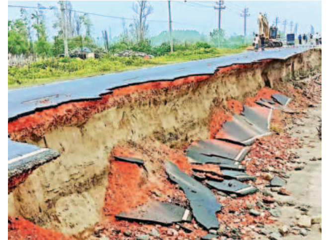
The erosion in some parts of the Marine Drive has taken a grave turn from Thursday, affecting at least 10 points in Teknaf. Around half of the 50-metre wide Marine Drive in west Mundardail area was washed away after geo tubes for protecting the road were torn apart by strong waves. PHOTO: STAR
