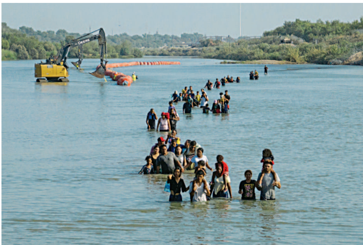
A caravan wades past a string of buoys, being constructed to deter migrants crossings through the Rio Grande river, as they look for an opening in the concertina wire to enter into Eagle Pass, Texas, US n Thursday.
