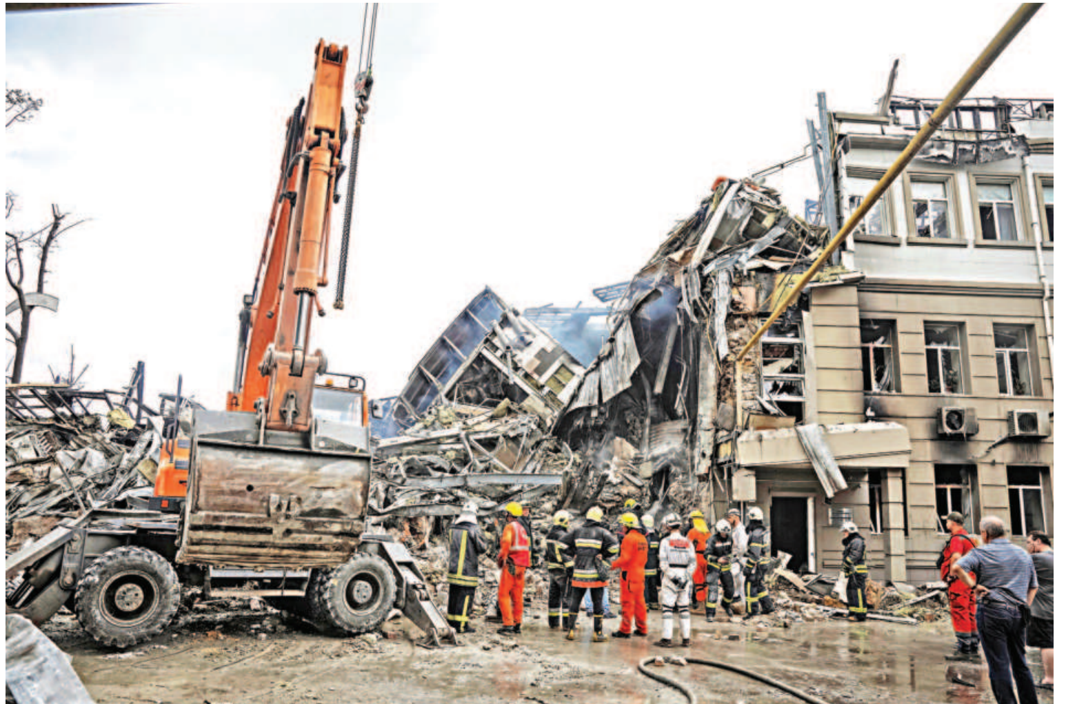
Rescuers work at a site of a building heavily damaged by a Russian missile attack, as Russia's attack on Ukraine continues, in central Odesa, Ukraine yesterday. PHOTO: REUTERS
