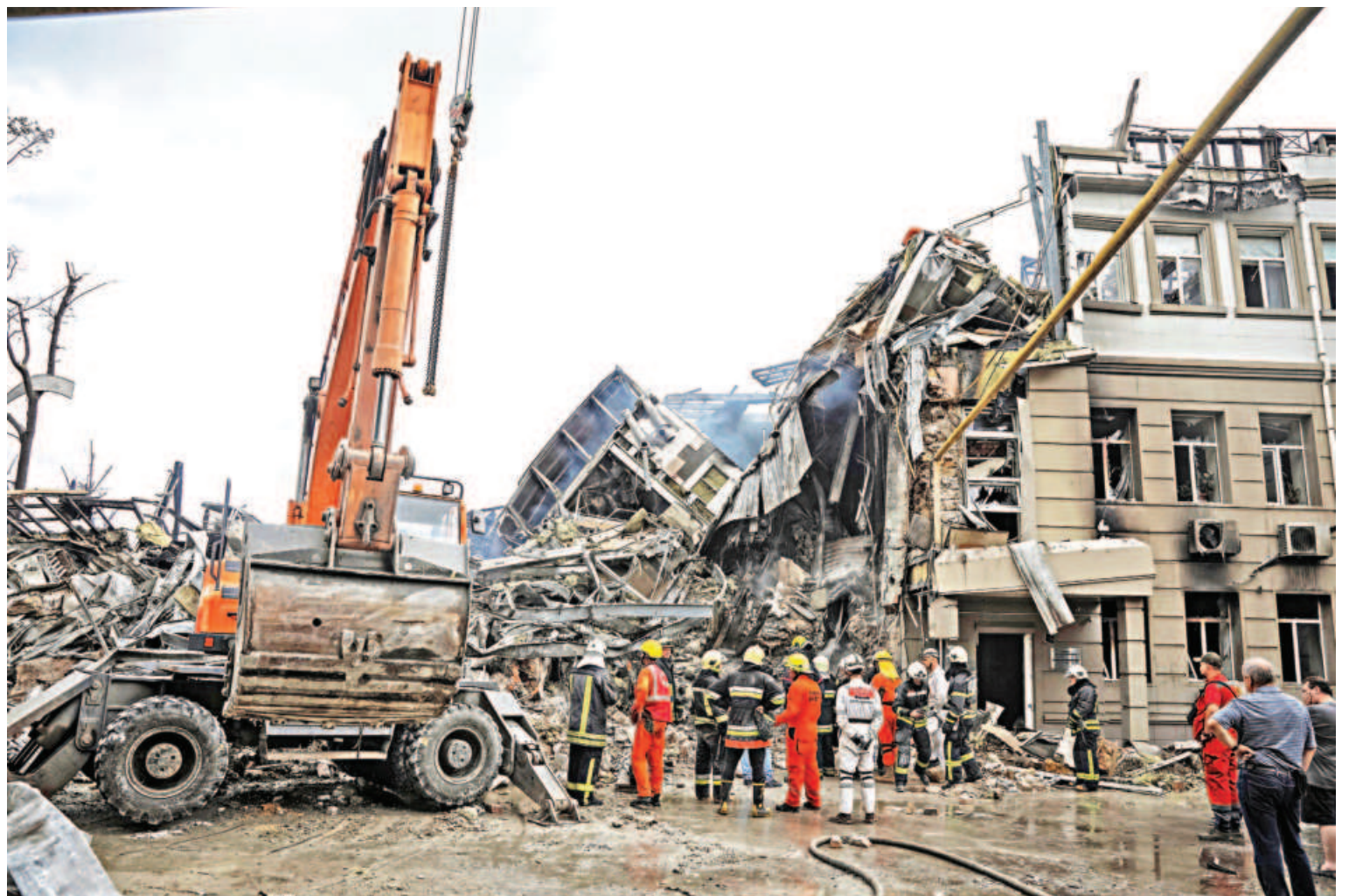
Rescuers work at a site of a building heavily damaged by a Russian missile attack, as Russia's attack on Ukraine continues, in central Odesa, Ukraine yesterday. PHOTO: REUTERS
