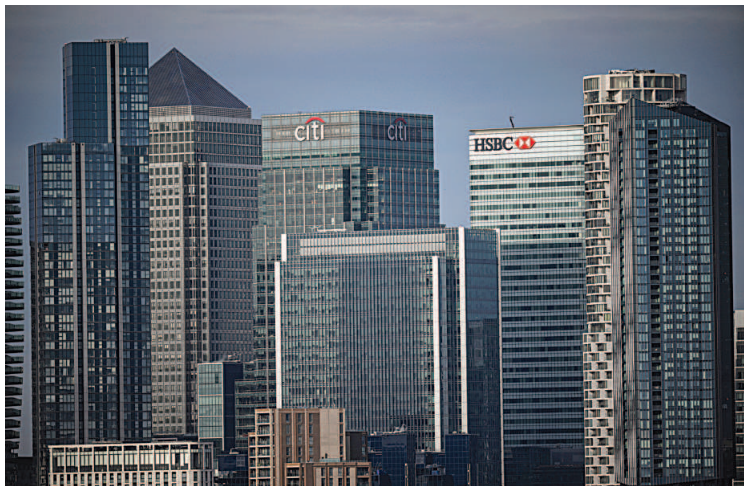
Bank buildings are seen in Canary Wharf financial district in London. London has been pushing a "Global Britain" strategy since formally severing nearly 50 years of ties with its nearest neighbours in the European Union three years ago.
