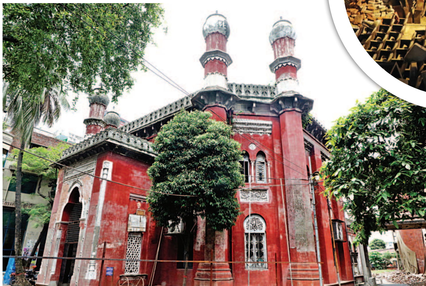
Over time, the historic Lalkuthi lost its former glory and faded into a state of neglect.
