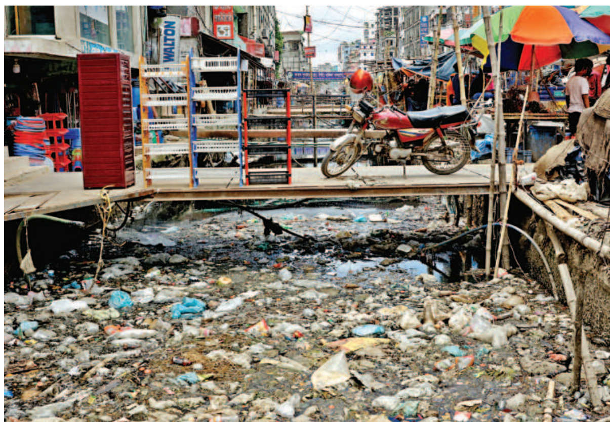
The Gabindapur canal in the capital's Shonirakhra remains choked with plastic waste. Local have set up makeshift bridges on it to cross over. Meanwhile, the platforms are also being used as a parking and storage space.
