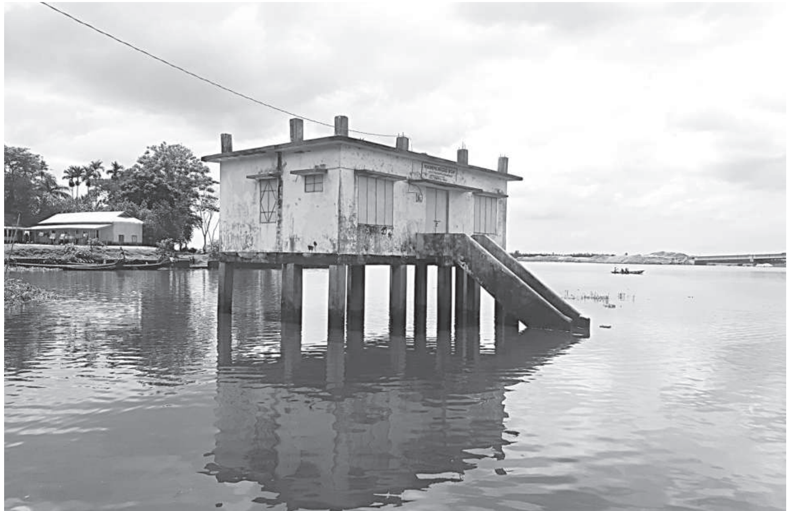
Madhabpasha Community Clinic remains surrounded by water at least four months a year. Due to a lack of accessibility, locals are often unable to seek medical help. This photo was taken recently.
