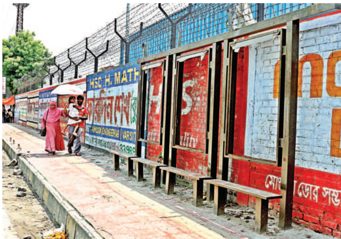
Shielding themselves from the scorching sun with an umbrella, a family walks past a structure that used to be a passenger shed near the Kamalapur container depot yesterday. Due to a lack of maintenance, the ceiling of this shed fell off a long time ago, and now just the rusted frame remains in place, unable to serve its purpose.
