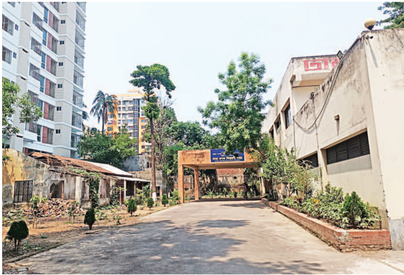
The abandoned compound of the Mosquito Control Department, where an empty two-storey building and neglected tin sheds stand in eerie stillness. Water accumulates after every rainfall, creating a breeding ground for mosquitoes, meaning the very place set-up to combat these disease-carrying insects inadvertently fosters their proliferation. This photo was taken recently in Old Dhaka's Dhakeshwari area.
