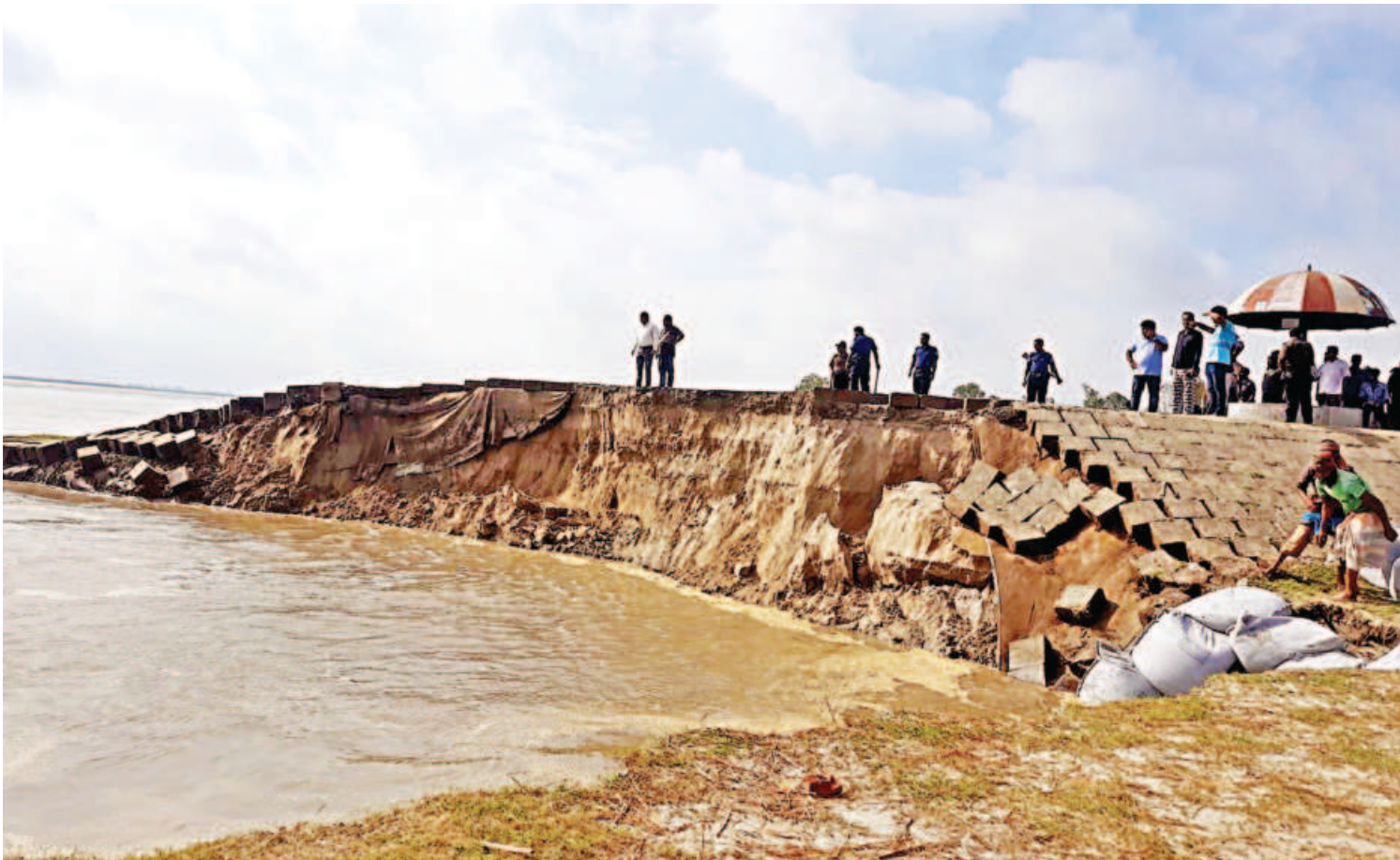
The Jamuna has eroded away a huge chunk of an embankment at Meghai Ghat in Sirajganj's Kazipur upazila. Bangladesh Water Development Board yesterday started dumping sandbags to curb further erosion. Locals are worried that a breach of the embankment will leave many key installations, including the Kazipur Police Station, at risk.
