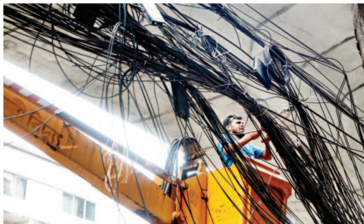
A city corporation worker removing a tangled web of overhead cables, which has been a long-standing nuisance for Dhaka residents. The photo was taken in Paltan area yesterday.
