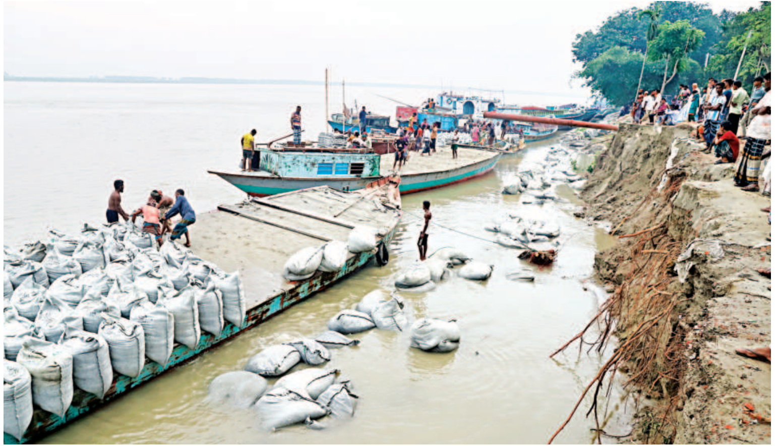
Water Development Board workers lining the Jamuna with geo bags -- made of woven polyester and polypropylene fabrics and filled with sand and/or soil to build shore-protection structures -- to stop river erosion at Chitulia village and beyond in Tangail's Bhuapur upazila. According to locals, erosion has been going on for around two months. The photo was taken recently.
