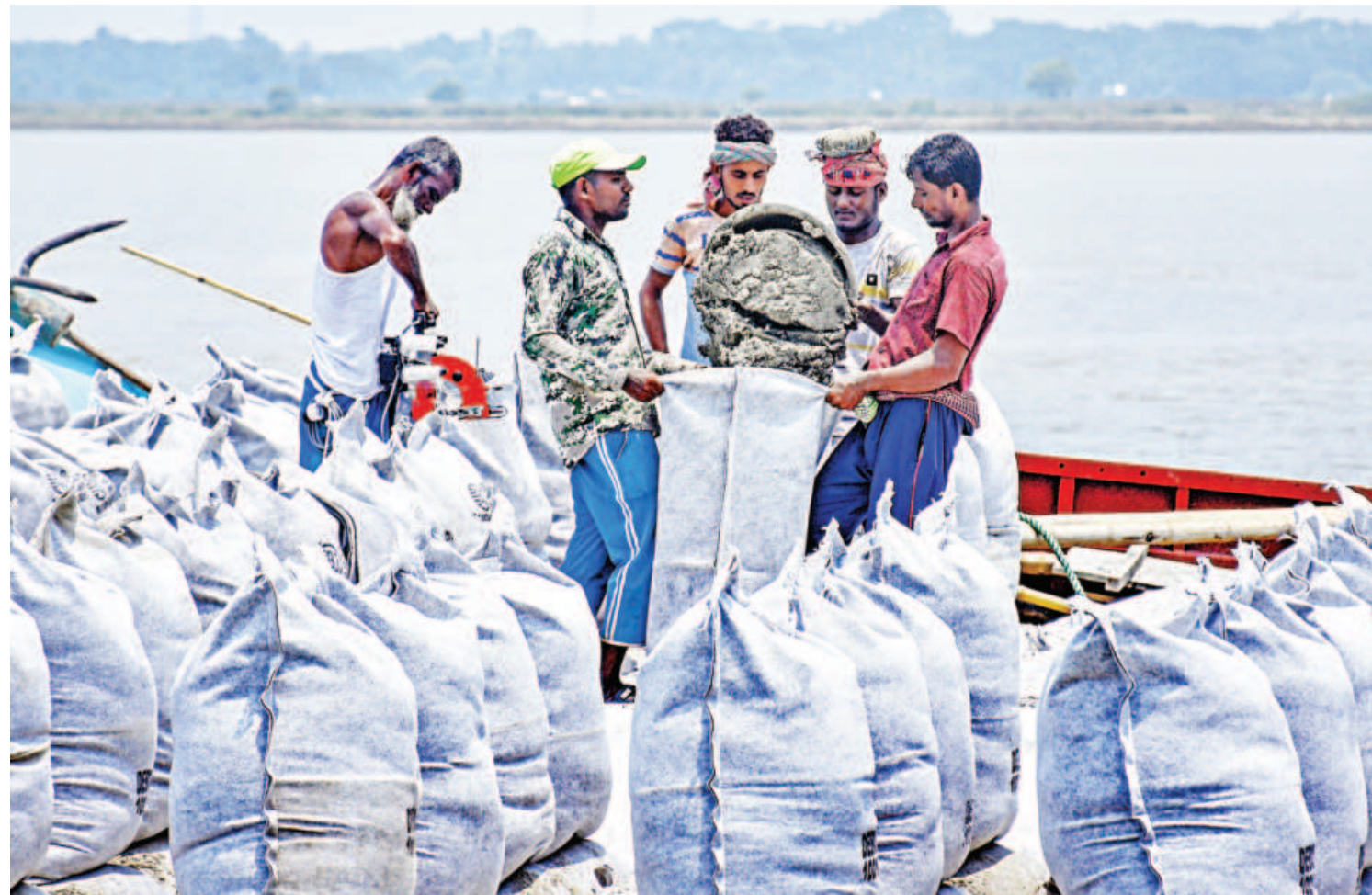
Day labourers fill up sand bags on board a trawler on the Rupsa river in Khulna. The bags are used to protect embankments from erosion. In Bangladesh, workers are going through a difficult time as their wage growth has not gone up in line with surging inflation. The photo was taken yesterday.
