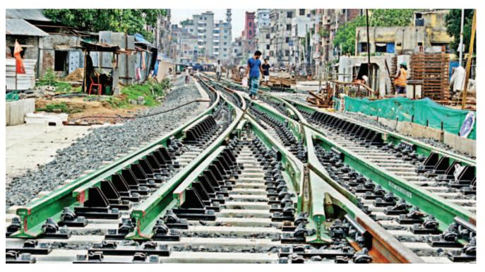
Bangladesh Railway is laying three new dual-gauge lines from the capital's Kamalapur to Gendaria under the Padma Bridge Rail Link Project. The lines will be used for the Dhaka-Narayangani and Dhaka-Jashore rail operations. With the work for laying one of the lines already completed, rail services on Dhaka-Narayangani route are expected to resume soon. The photo was taken in the capital's Titipara area recently.
