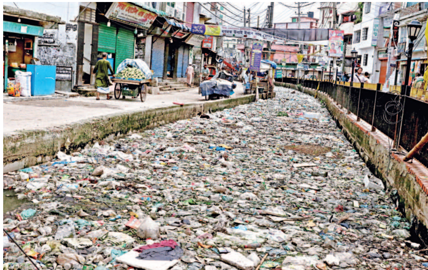
The Kutubkhali canal is clogged with waste in Madrasa Road area of the capital's Dakshin Jatrabari. Many areas in the city remain waterlogged after rain as clogged canals cannot drain water. Uncleaned water bodies also become safe breeding grounds for mosquitoes. The photo was taken on Sunday.
