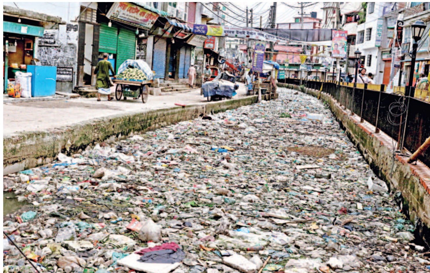
The Kutubkhali canal is clogged with waste in Madrasa Road area of the capital's Dakshin Jatrabari. Many areas in the city remain waterlogged after rain as clogged canals cannot drain water. Uncleaned water bodies also become safe breeding grounds for mosquitoes. The photo was taken on Sunday.
