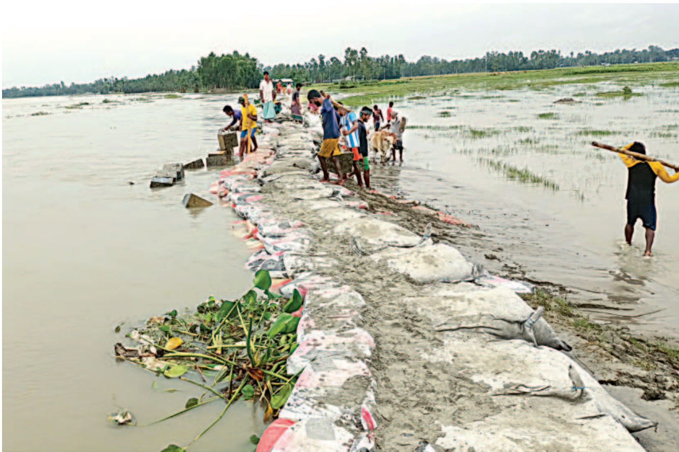
Workers of Bangladesh Water Development Board dump concrete blocks and sandbags on a road along the Dudhkumar river in Pateshwari area of Kurigram's Nageshwari upazila yesterday. The river has been swelling due to rain and onrush of water from upstream and threatening to flood farmland and villages on the right.
