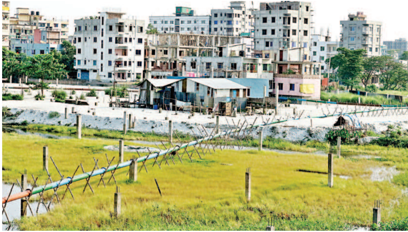
People use illegally dredged silt from rivers to fill low-lying areas and floodplains so that those can be turned into housing plots. They use pipes like the one in the photo to conduct their illegal activity on an industrial scale. The photo was taken at Trimohani in the capital.
