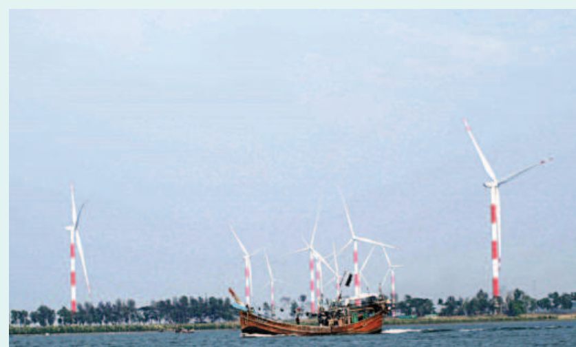
Construction of a 60-megawatt wind power plant is going on in Khurushkul of Cox's Bazar. The plant has recently started producing power on a trial basis. The photo was taken last month.
