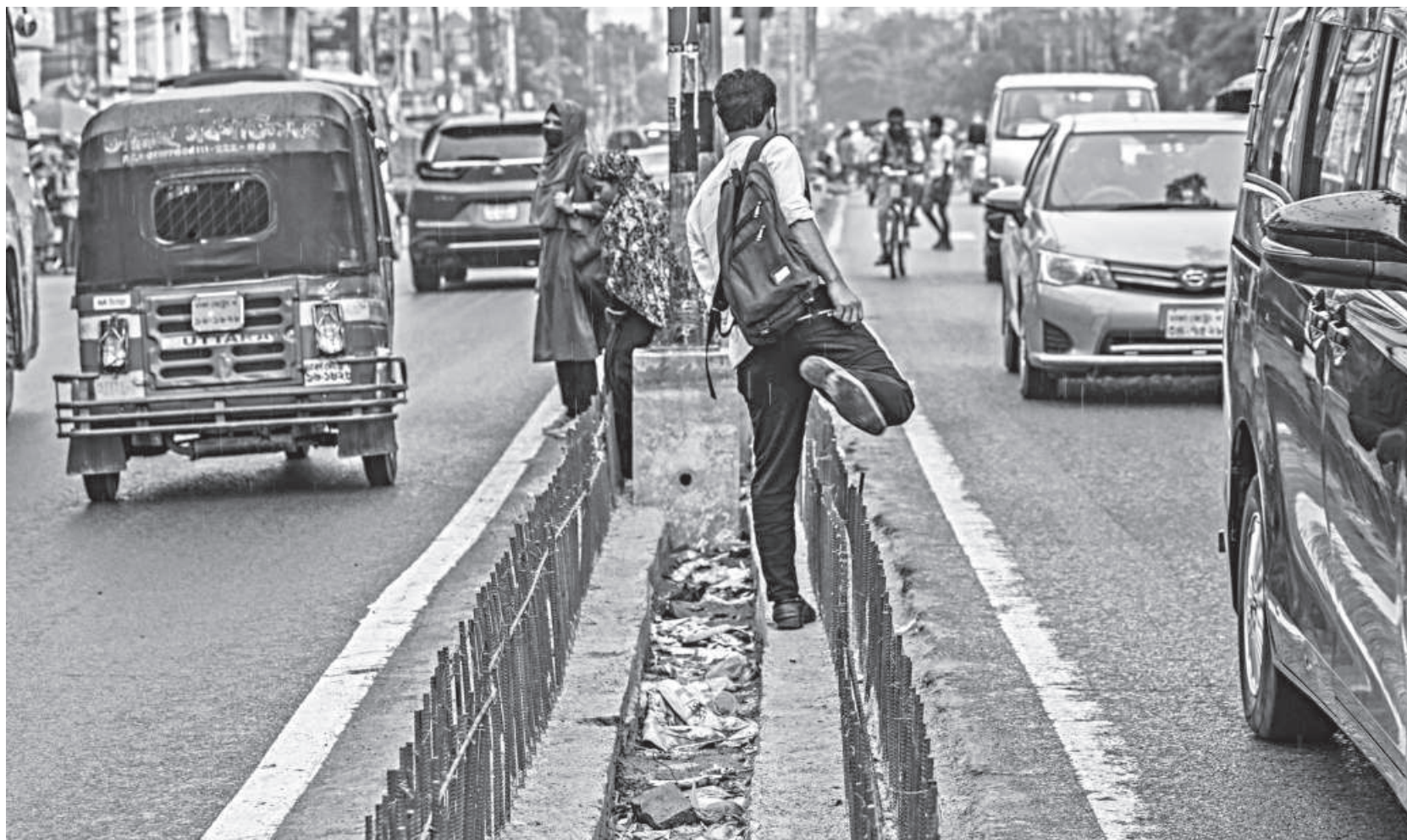
With speeding vehicles coming from both directions and no foot-over bridge nearby, pedestrians have to leap over the iron rods on the under-construction median to cross the capital's Satmasjid Road. This photo was taken yesterday near Jigatola intersection.
