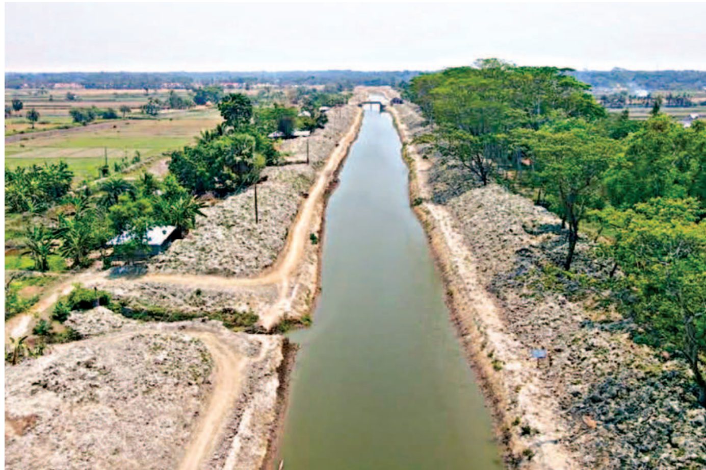
A re-excavated canal, known as Mora Posur, gets a new lease of life. Seven such canals, including this one, were re-excavated in Betaga union of Bagerhat's Fakirhat. Now farmers are getting irrigation water from them. The photo was taken in Betaga village recently.
