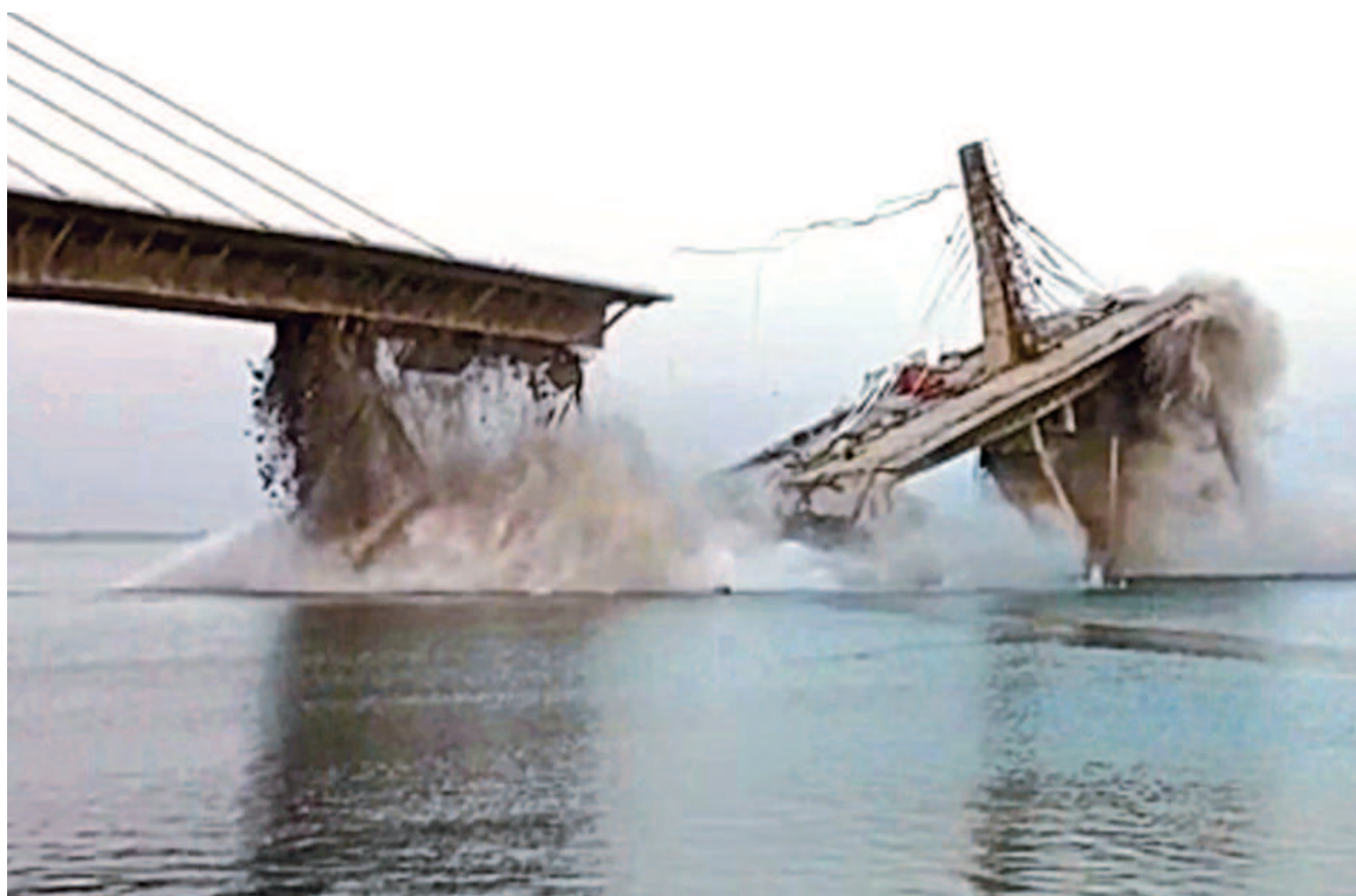
This photo taken on Sunday and released yesterday, shows an under construction bridge collapsing into the river Ganges in Bhagalpur district in India's eastern state of Bihar. Eight men were on the bridge at the time of its collapse on Sunday, with one guard reported missing.
