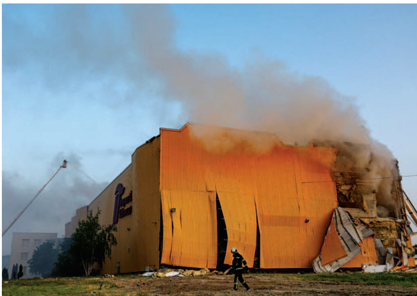
A firefighter works at a site of a tobacco factory damaged during Russian suicide drone strike, amid Russia's attack on Ukraine, in Kyiv yesterday.
