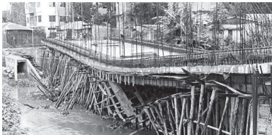
Even after a year, the bridge over Louhajang river in west Tangail is in its worst shape due to the delay in the reconstruction works. Earlier, the bridge collapsed after half its construction was completed.
