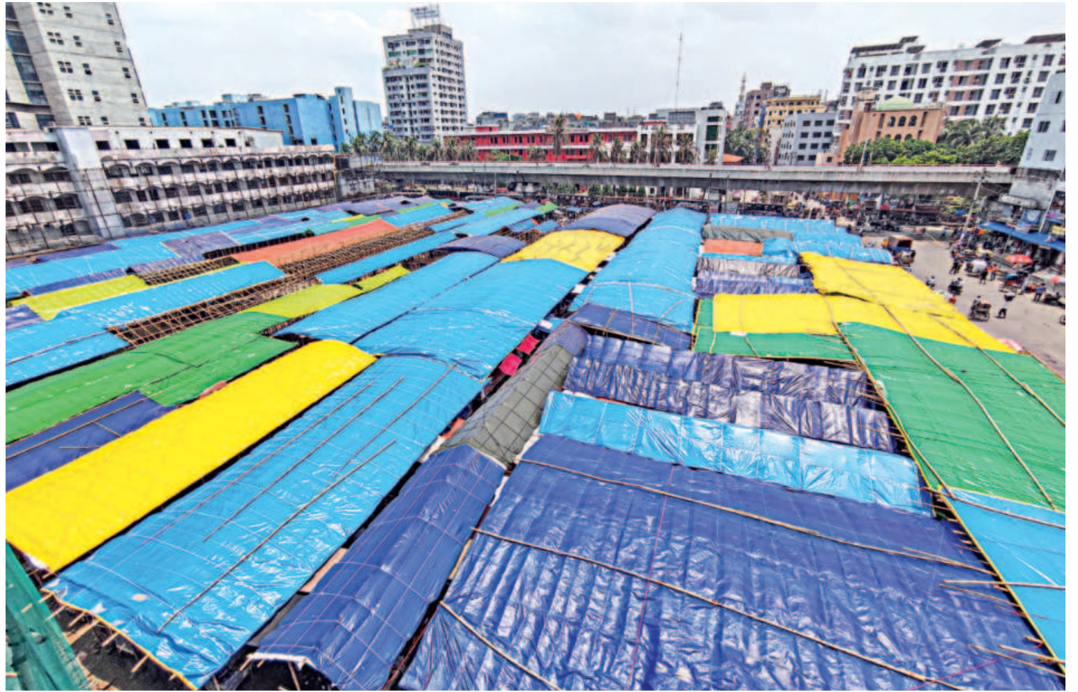
Traders continue their business at a makeshift market, which once used to be the bustling Bangabazar Shopping Complex. After a massive fire burnt it down last month, they set up cots at the site and covered those with colourful plastic sheets to protect them from rain. This photo was taken yesterday.
