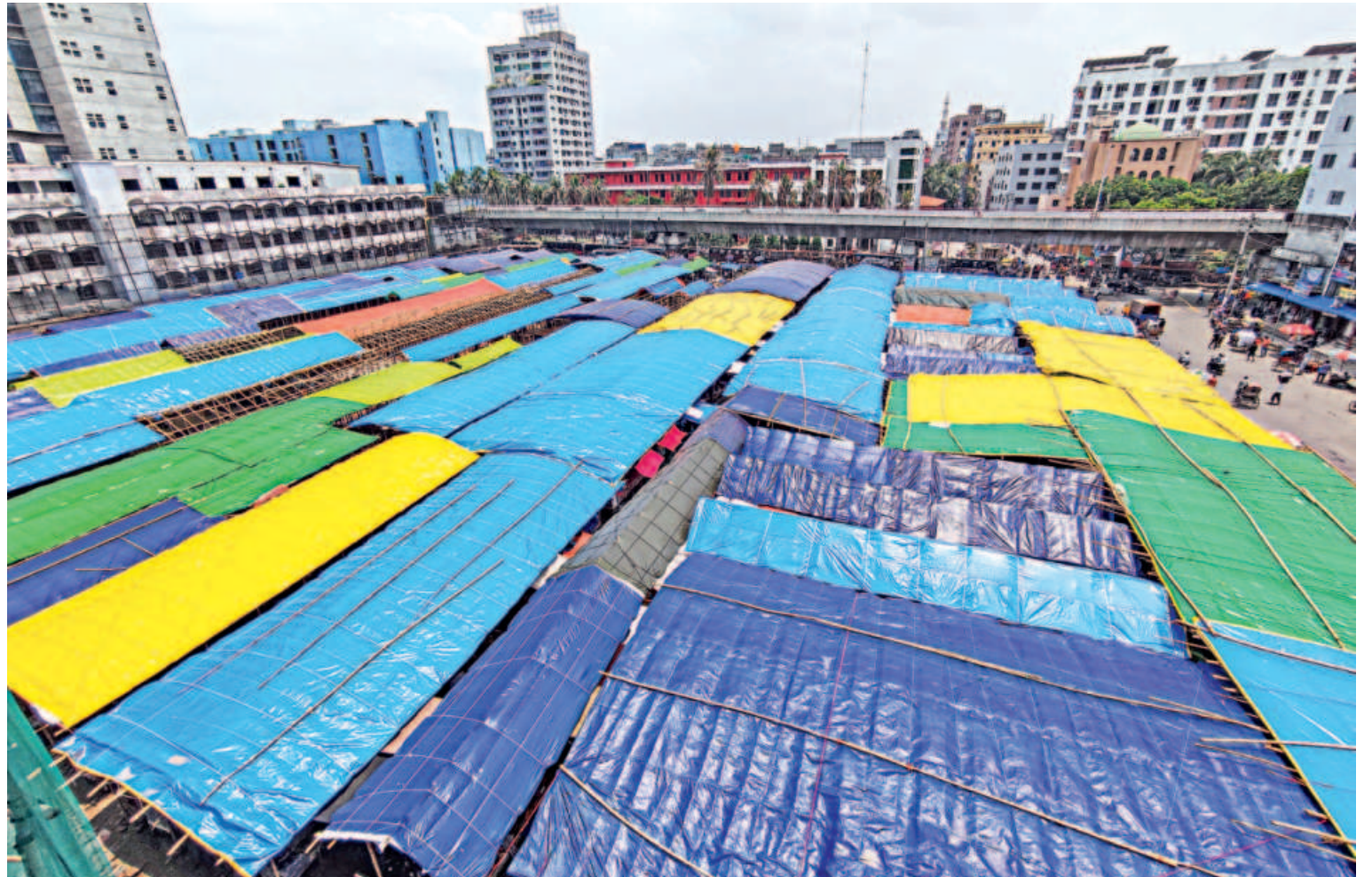
Traders continue their business at a makeshift market, which once used to be the bustling Bangabazar Shopping Complex. After a massive fire burnt it down last month, they set up cots at the site and covered those with colourful plastic sheets to protect them from rain. This photo was taken yesterday.
