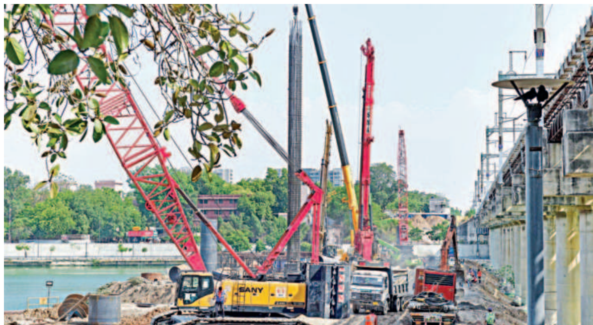
Heavy machineries are seen installed at the construction site of the Mumbai-Ahmedabad high-speed rail corridor across Sabarmati river in Ahmedabad on May 18. PHOTO: AFP
