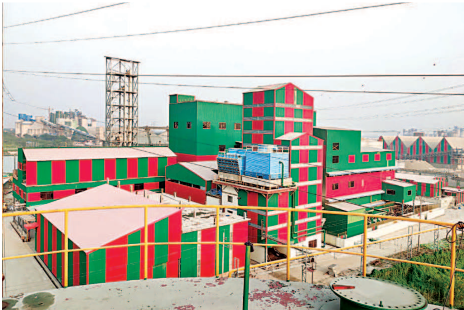
The view of a factory of Delta Agro Food Industries, a joint venture of Seacom Group and Samuda Group, in Narayanganj. The plant was up at an investment of more than Tk 1,200 crore one and a half years ago, but it has not been able to go into production due to a lack of gas connection.
