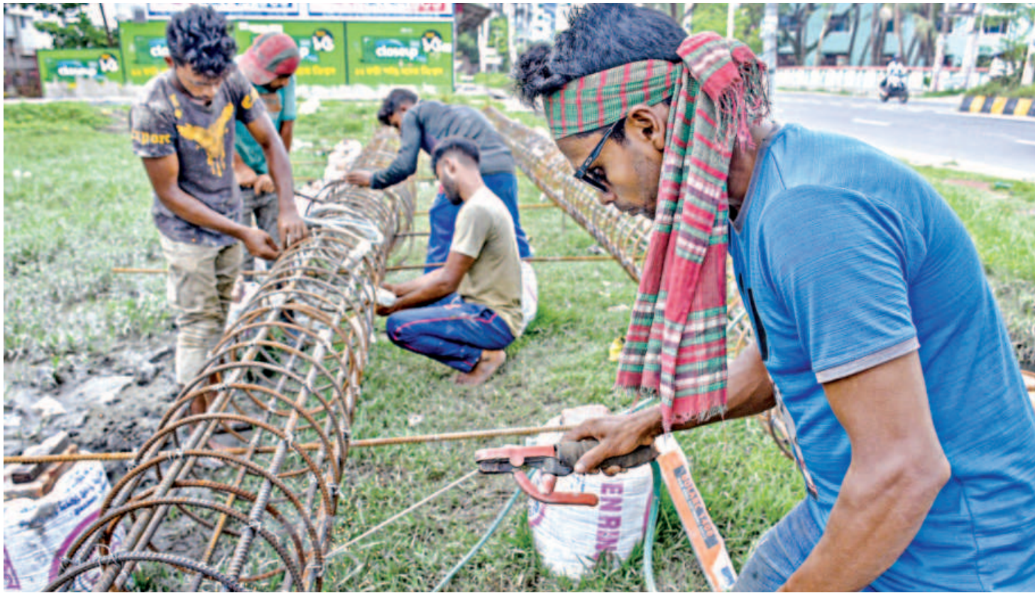
Workers build cages bending and welding together steel rods for piling foundations into the ground. The piles are built under different structures to transfer loads from the structures to the ground, helping to support them. Five workers can prepare anywhere from five to six cages in a day, earning Tk 600 each. The photo was taken from Khulna city on Sunday.
