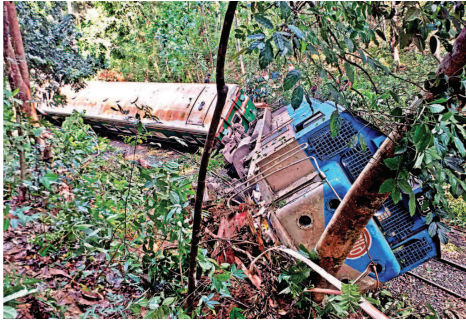
Sylhet's rail link with Dhaka and Chattogram was suspended for 15 hours after parts of a train derailed at Lawachhara National Park in Moulvibazar's Sreemangal upazila early yesterday.
